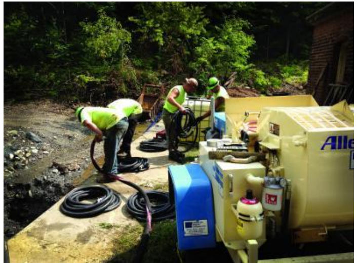
The minimal staging area required made CCCP technology an ideal solution for this project.
